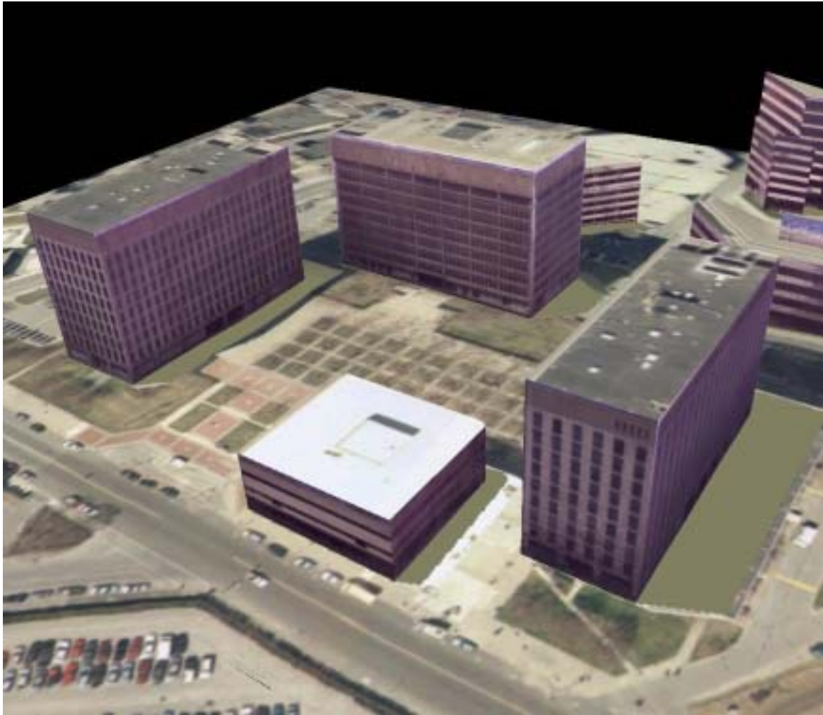
Figure 1-4: Goal of the city project. Rendering from an idealized model built with human input.
