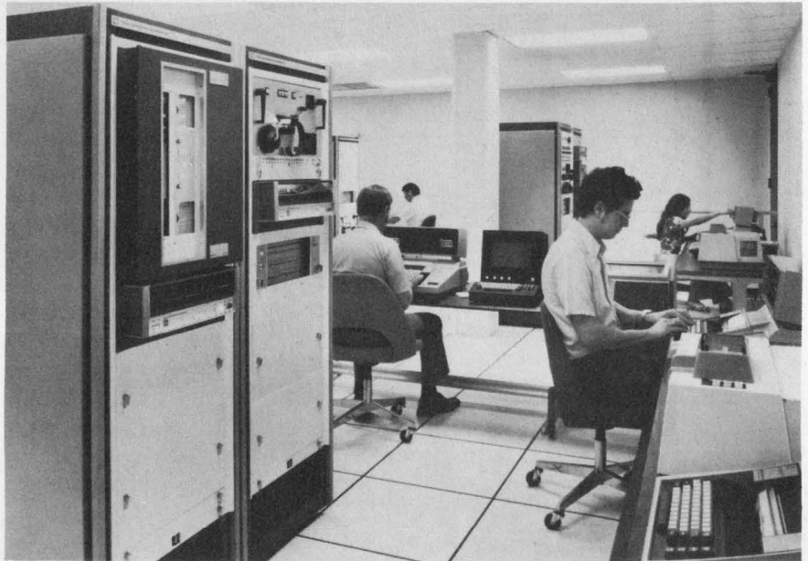
Multi-terminal 980A System
